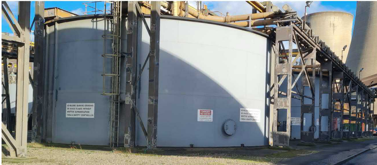
Plate 7.1 - Example of an Existing Tank
