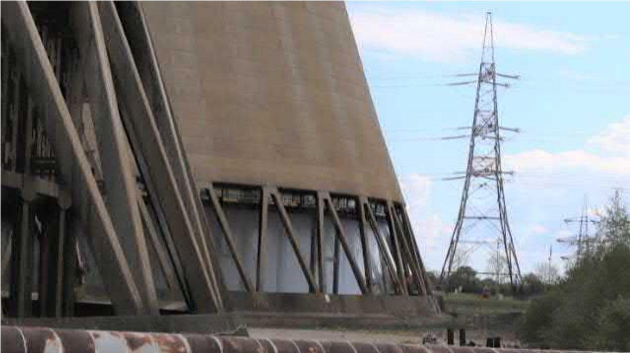
Plate 5.11 - Example of the Cooling Water Reservoirs
